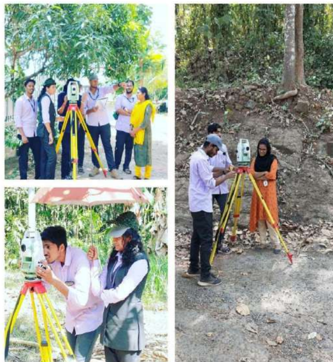
Figure 2.2.1.m Images taken during rebuild Kerala works
